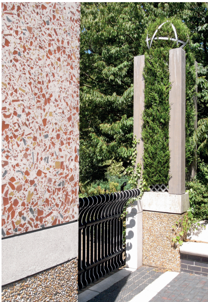
The 'folly' of the 'grown' Serliana lies across a Badger-Gate to hold such invaders at bay. The House-column stratifies into Earth (gravel-crete), Water (limestone-crete), and the Light, or Fire of 'exploding' Blitzcrete.
